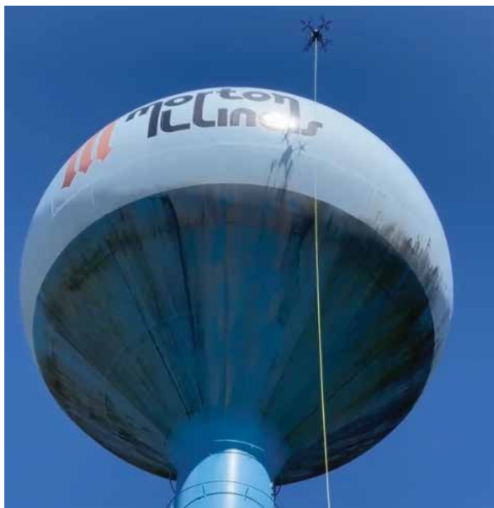
Apellix builds tethered drones that carry a pressure-wash wand and spray tips up the side of a tank.
